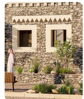
4 Landscape strip partially concealing the elevated windows of the ground floor
