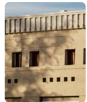
4 Horizontal banding with layering of bricks
