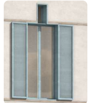
2 Integrated high level vents
