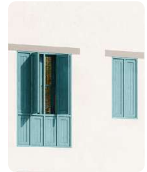
2 Shuttered window with expressed lintel
