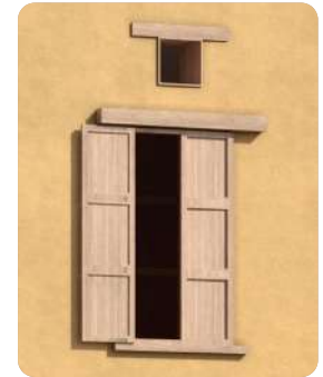
2 Larger timber framed and shuttered windows with high level vents.
