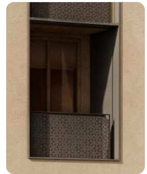
3 Introduction of perforated metal shading screens.
