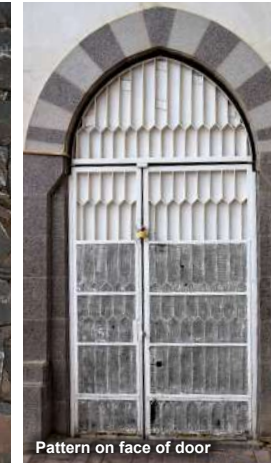
Pattern on face of door
