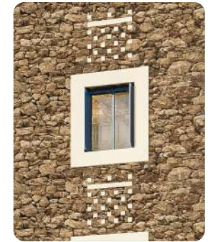
2 Punched window openings with colored timber shutters, white surrounds and pattern highlights
