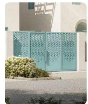
4 Vehicle gates integrated in boundary wall.
