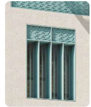
2 Windows: deep set with integrated overpanels
