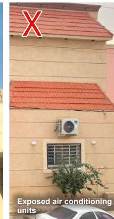
Exposed air conditioning units
