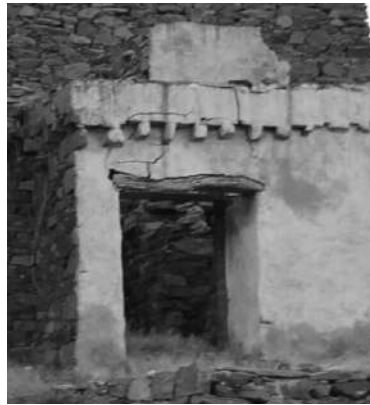
Parapet with crenelations
