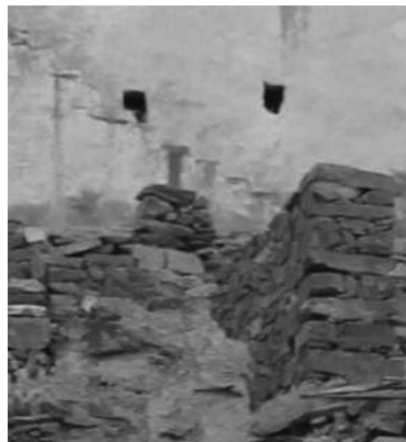
Defense / ventilation openings
