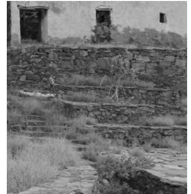
Terraces and compound walls
