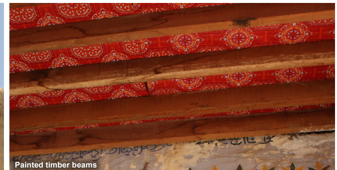
Painted timber beams
